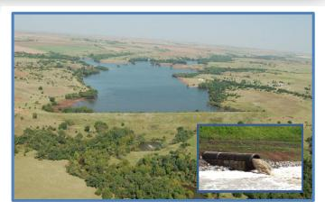
A series of flood control dams constructed in a watershed impound water from heavy rainfall events and slowly release it through a pipe in the dam over a period of days or weeks. This reduces flooding downstream.
